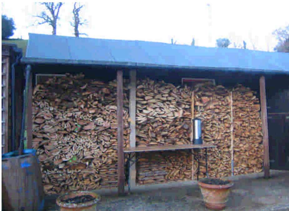
Figure 5: Boiler house and woodfuel store
