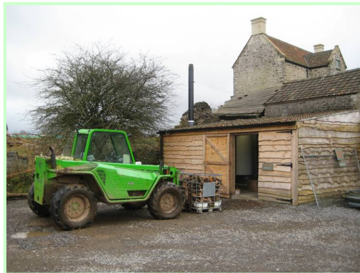
The boiler house and flue. A telehandler is used to move baskets of logs.
