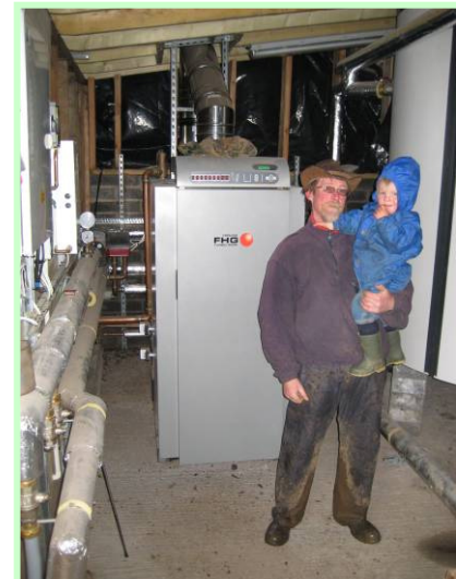
Andrew Wear and his son Seth with their Frolina 70 kW log boiler
