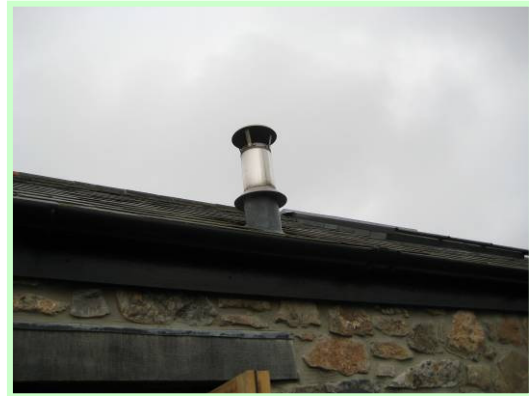
As long as the boiler is functioning properly no smoke is produced from the flue.
