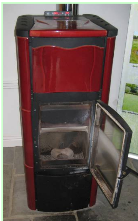
The stove needs vacuuming out to remove dust every week and de-ashing every month.
