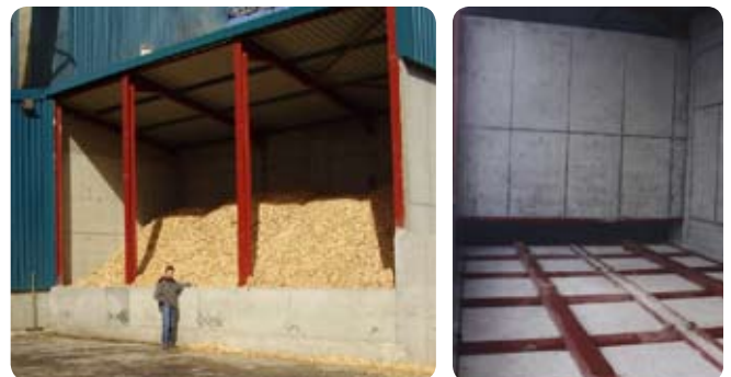
The 280m 3 fuel store at Strabane Mills with moving floor detail
