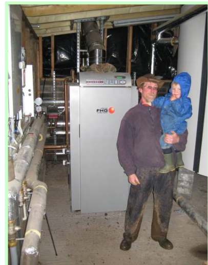
Andrew Wear and his son Seth with their Froling 70 kW log boiler
