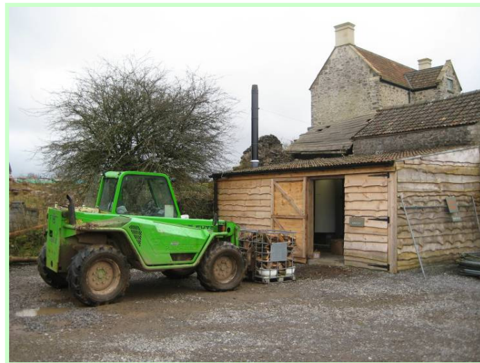
The boiler house and flue. A telehandler is used to move baskets of logs.
