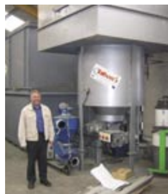
Left: waste wood is cheapest fuel. Right: Talbot's has a 250kW unit.
