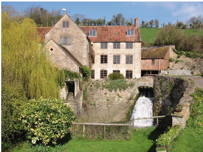
Top: N Yorks farmers Ann and David Kiely are converting a 1750s water mill to produce 55kW/hr. Above left and right: Brian and Alison Shingler installed a new turbine at Gants Mill, Somerset. It produces 12kW/hr.
