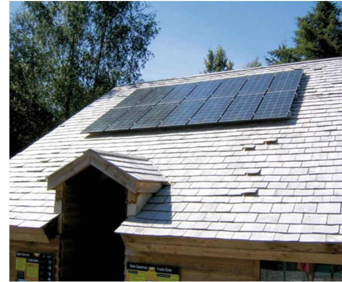
Photo-voltaic cells are available in panels (left) and individual replacement tiles (above).
