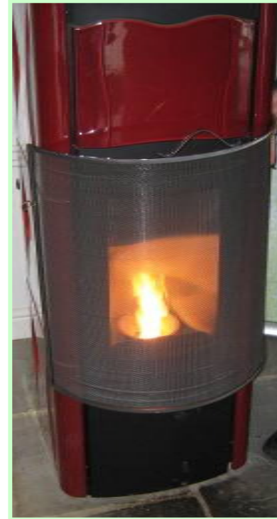
The stove front can get hot so there is a fire guard that can be used as a safety feature.
