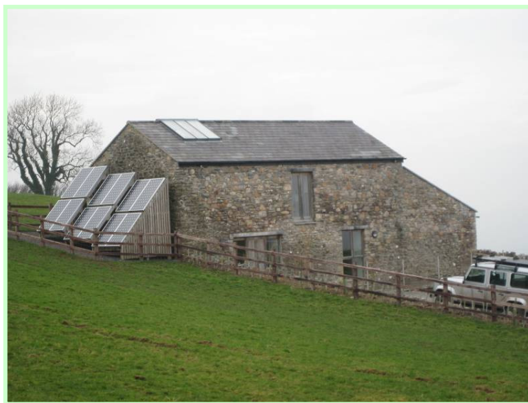
Wills Barn is situated in the Mendip Hills above Chew Valley Lake. The photovoltaic array is on the left of the building facing due south.
